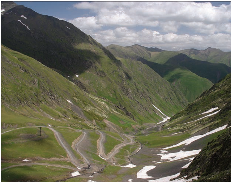
Road from Abano Pass
