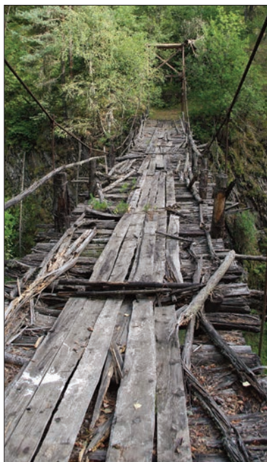
Old bridge on Omalo–Shenako route
